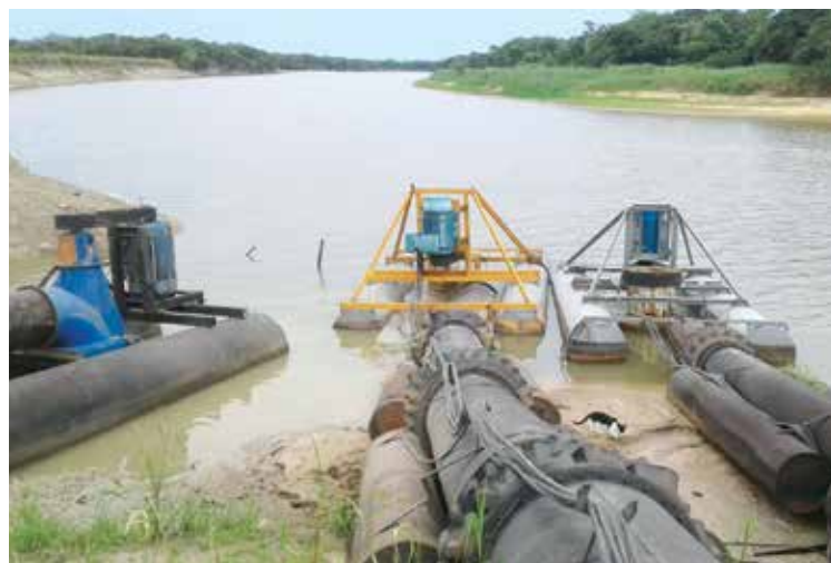
Pontoon-mounted pumps photographed in 2019 on Paraguay's Tobicuary River, where government inspectors say rice growers were extracting water for irrigation without permission. (Photo by Mades)
